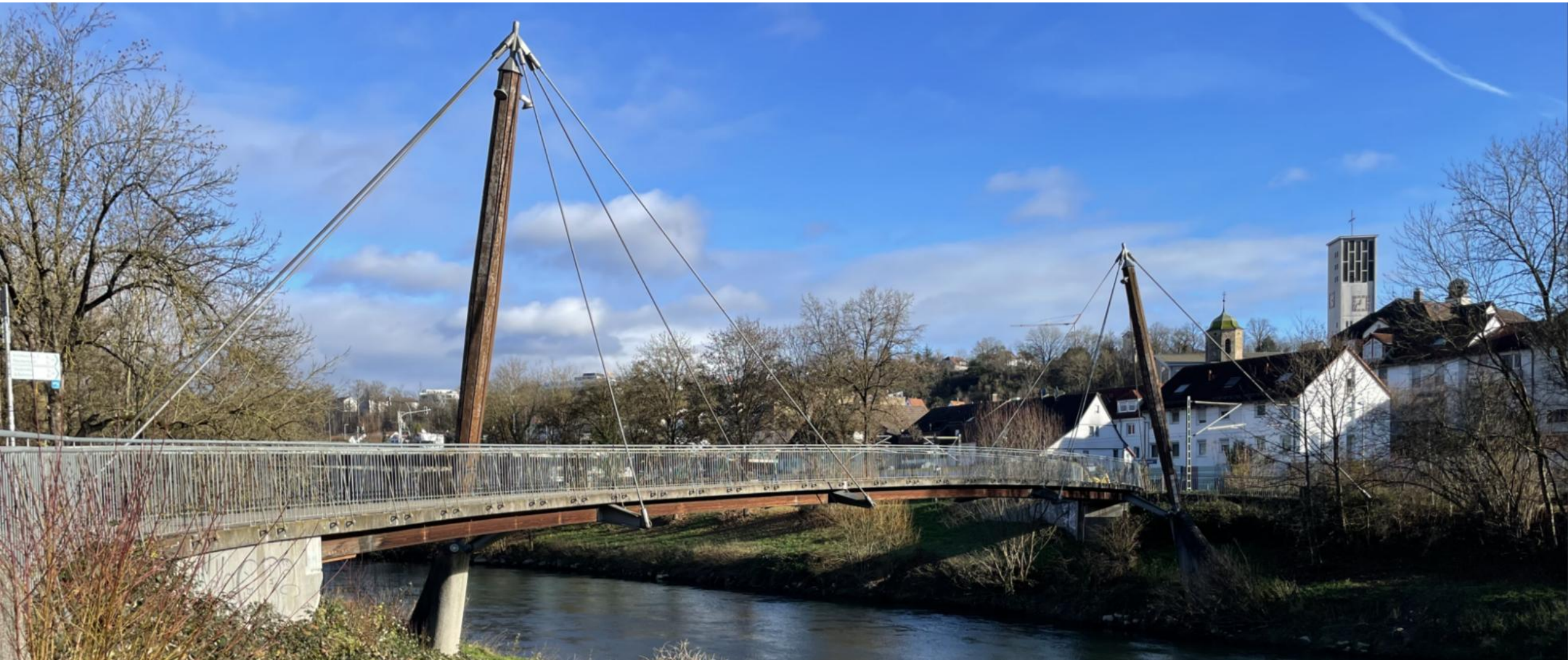
Bridge Wernau from 1989, DE
